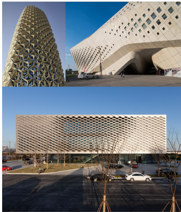
Figure 2: Recent examples of facades that follow a module-based approach. a. Al Bahar Towers, AEDAS, Image Credit: AEDAS; b. Nanjing International Youth Culture Centre, Zaha Hadid Architects, Image Credit: Khoo Guo Jie; c. Nantong Urban Planning Museum, Henn Architekten, Image Credit: Bartosz Kolonko/HENN
